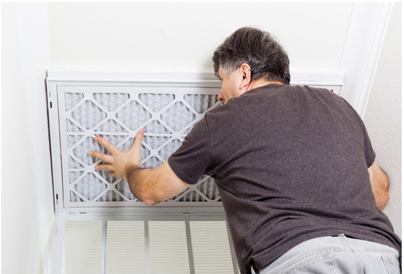
Image: HVAC filter installation © Borealis
