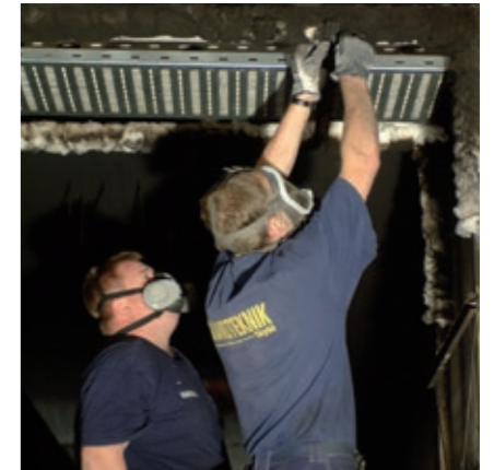
Preparation for large scale fire test
