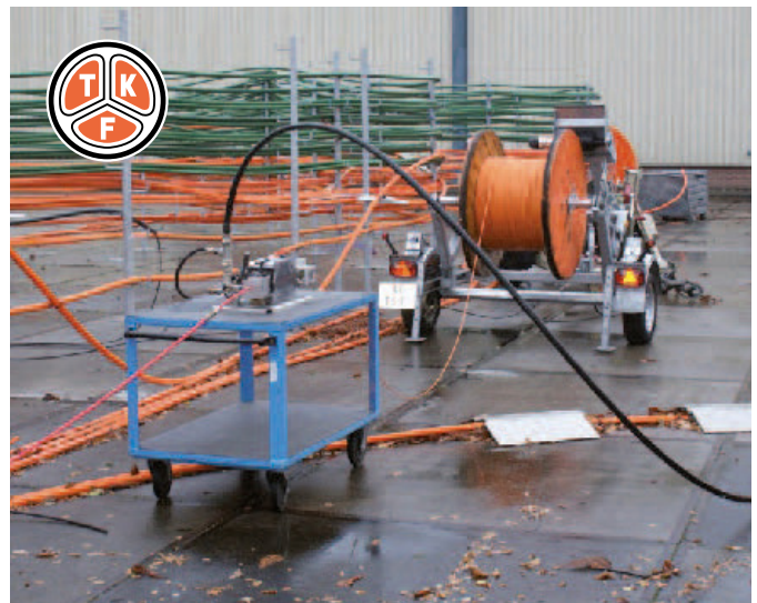
Test circuit for blown cable installation at TKF site
