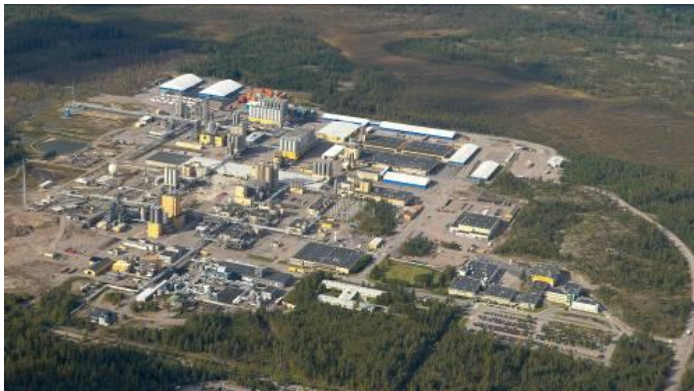
Borealis polyolefin plant in Porvoo, Finland
