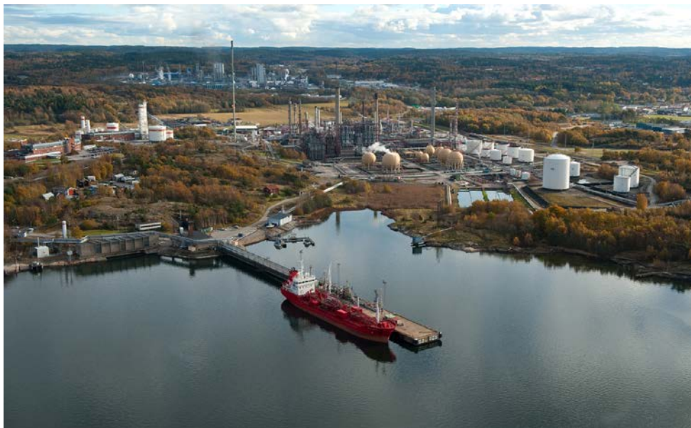
Borealis cracker plant in Stenungsund, Sweden.
