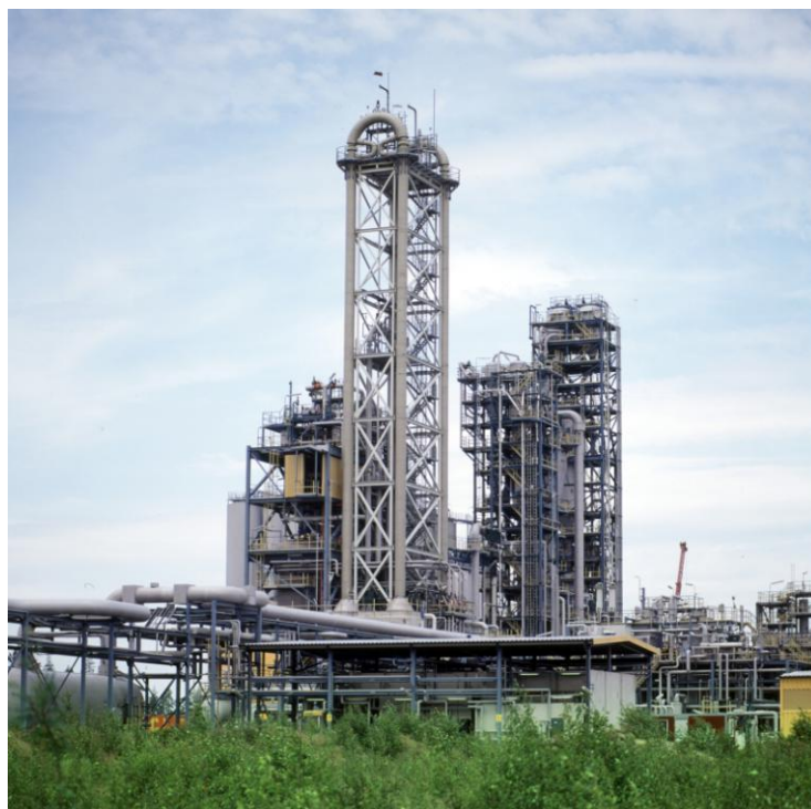
Photo: Borealis Borstar PE2 plant in Porvoo, Finland. © Borealis
