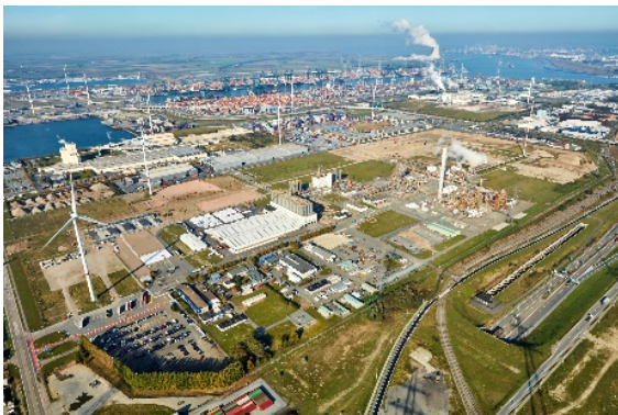
Photo: Aerial view of the Borealis production site in Kallo, Belgium.
