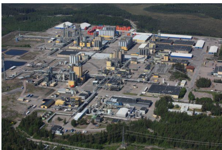
Photo: Borealis announces it is investing EUR 17.6 million in a new Regenerative Thermal Oxidizer (RTO) for its polyolefins plants in Porvoo, Finland.
